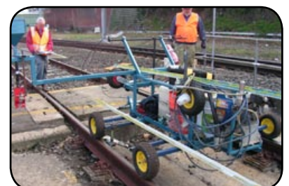
13 kilometres of luminous low location line marking in just 6 days!
